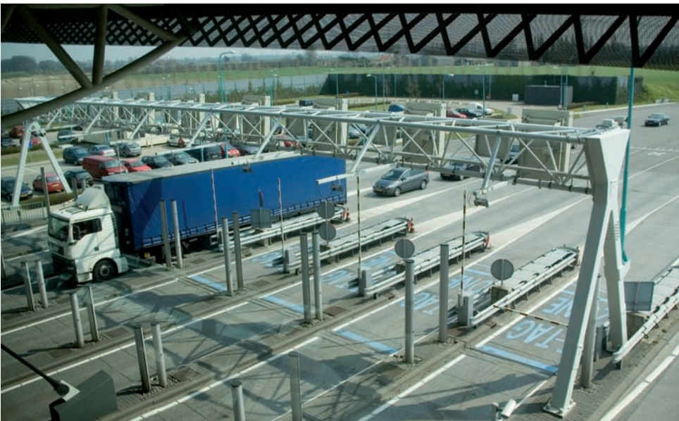
Westerscheldetunnel's toll plaza is 14 lanes wide, seven in each direction
